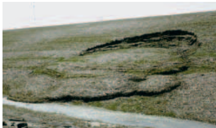
Figure 23 Earthflow This small, tongue-shaped mass movement occurred on a newly formed slope along a recently built highway.
