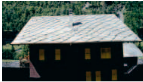
Figure 4 The roof on this house is made of slate. Slate is a metamorphic rock that forms from the sedimentary rock shale.
